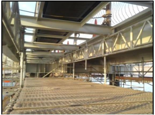
VIEW OF THE STRUCTURES AFTER MAINTENANCE (MARCH 2017)
