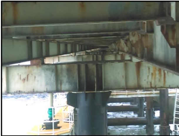
VIEW OF STRUCTURES BEFORE MAINTENANCE (JANUARY 2017)
